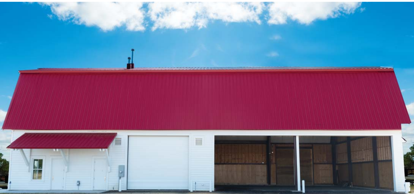
The new UGA-Tifton Campus Barn features three coiling steel roll-up doors for maximum space efficiency. Photos Courtesy of Charlie Fernandes.
